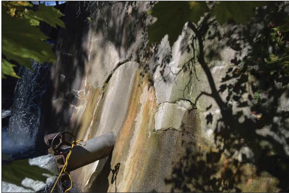
Photo # 16 – Cracks in Downstream Face Right Side
