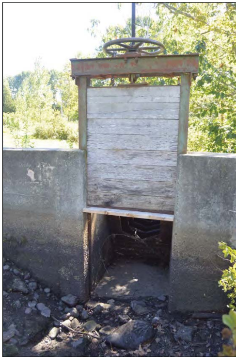
Photo # 6 – Fishway Control Gate on Left Abutment
