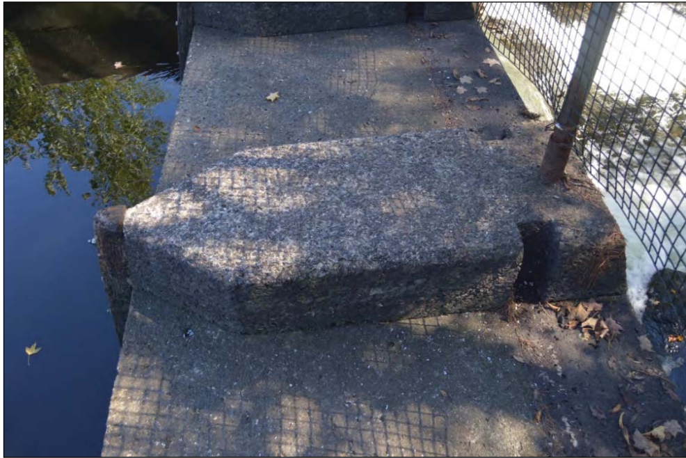
Photo 18 – Minor Concrete Erosion At Spillway Crest
