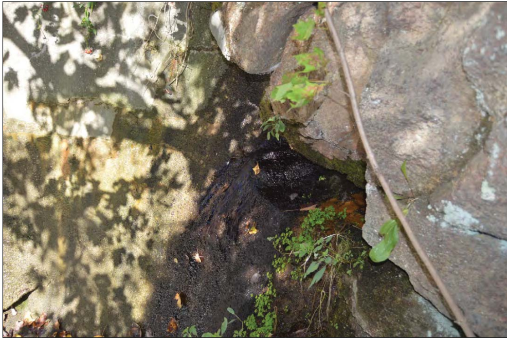
Photo #15 – Voids at Abutment near Penstock Ledge Interface
