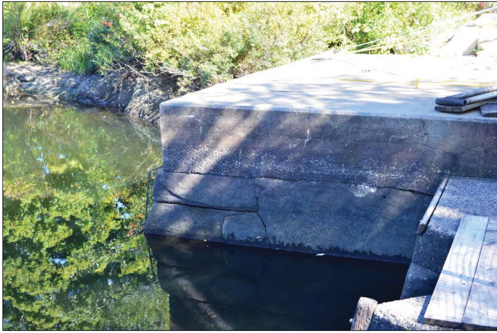
Photo #19 – Penstock Intake with Loss of Concrete
