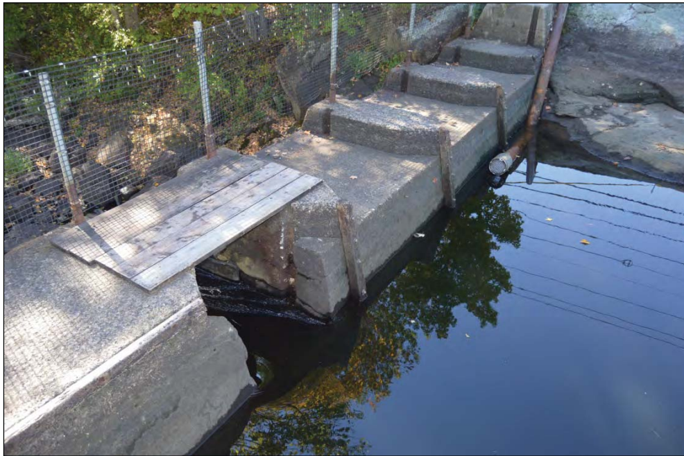
Photo #20 – Sluiceway with Concrete Cracking and Exposed Rocks
