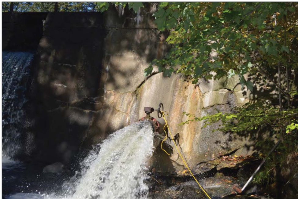
Photo #14 – Downstream View of Former Penstock with Low Level Outfall
